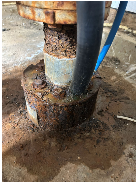
PHOTO 7 – View of Well #2.
