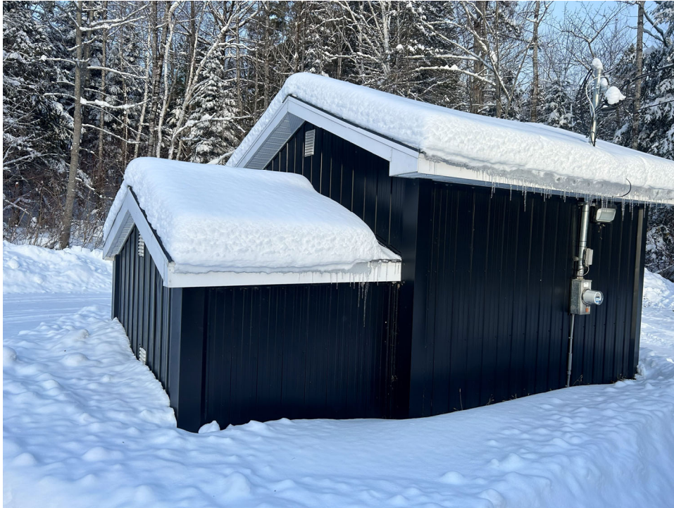
PHOTO 5 – View of Well #2 well house from east.
