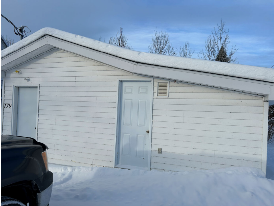
PHOTO 1 – View of Well #1 well house from east.
