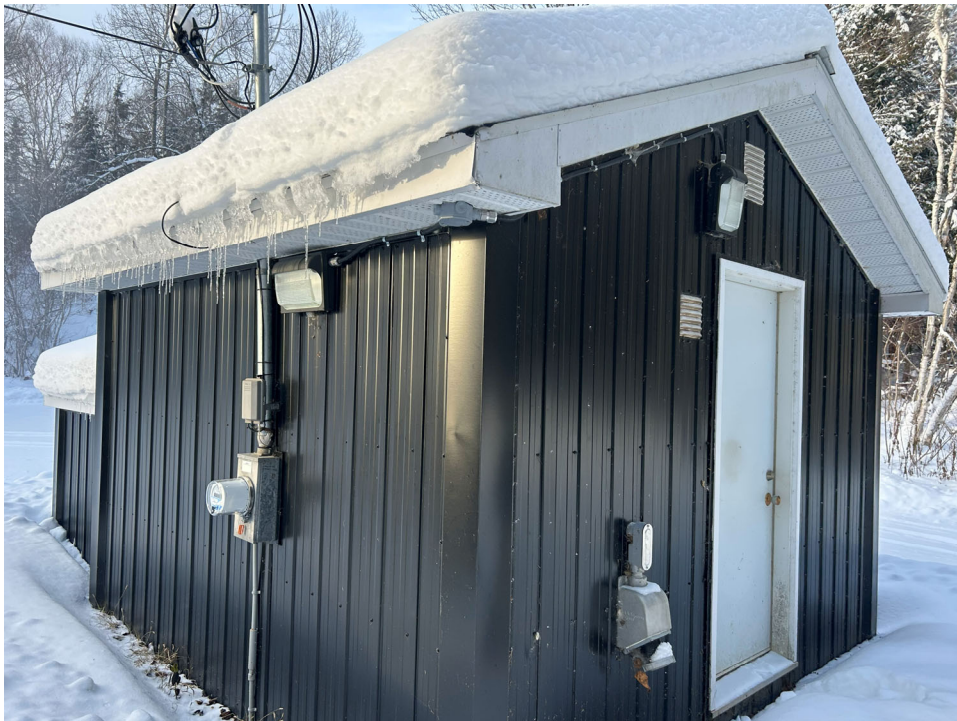
PHOTO 6 – View of Well #2 well house from north.
