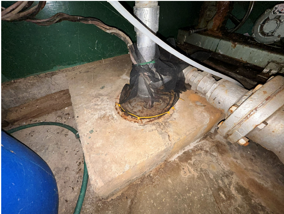
PHOTO 3 – View of Well #1.
