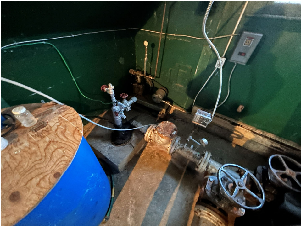
PHOTO 2 – View of Well #1.
